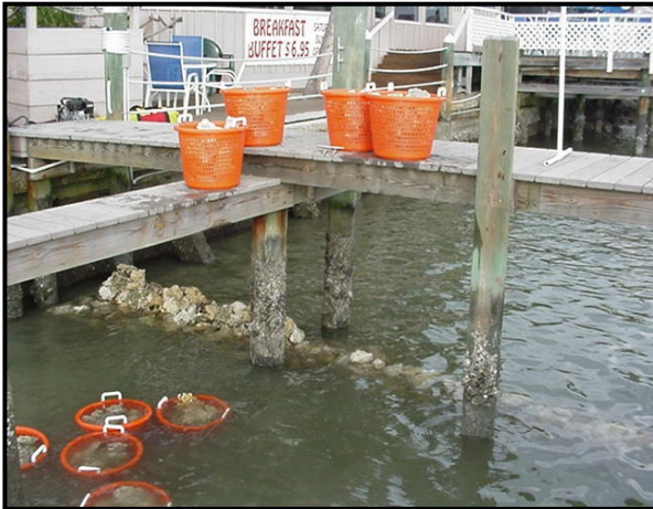
Placement of reef rock around dock ("The Pub" Reef Construction)
